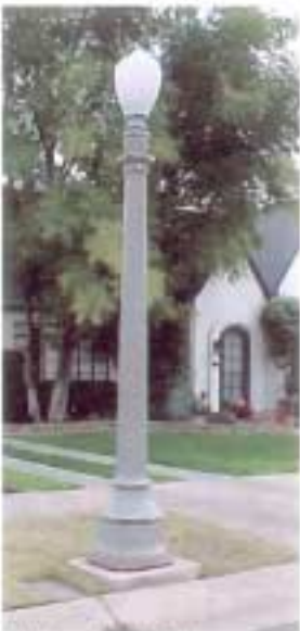
Photo 26. Replacement pole in Encanto-Palmcroat District.
