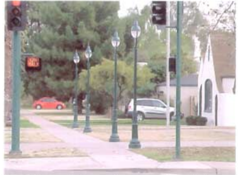
Photo 25. Restored fixtures are from City surplus yard and may have originally been used in City Parks. Inappropriate spacing and siting for streetlights.
