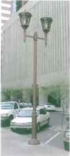
Photo 30. Copper Square streetlight.
