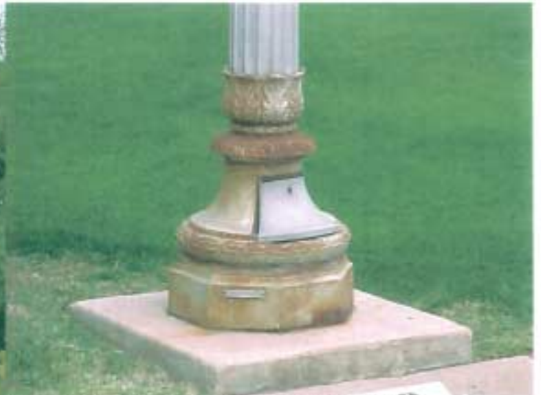
Photo 13. Historic metal poles are found only along Palmcroft Drive (NE, SE, SW), 11 th Ave. & Coronado.
