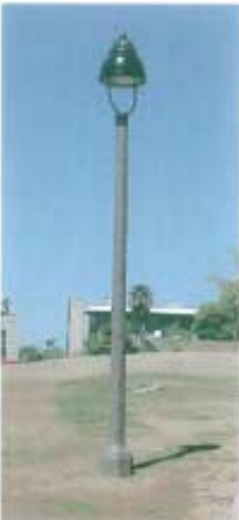
Photo 33. Modern cast concrete pole.
