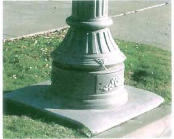
Photo 17. Installation similar to historic installation.
